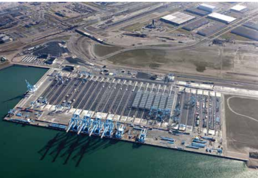
One of the best examples of current top-end automation is APMT Maasvlakte II
