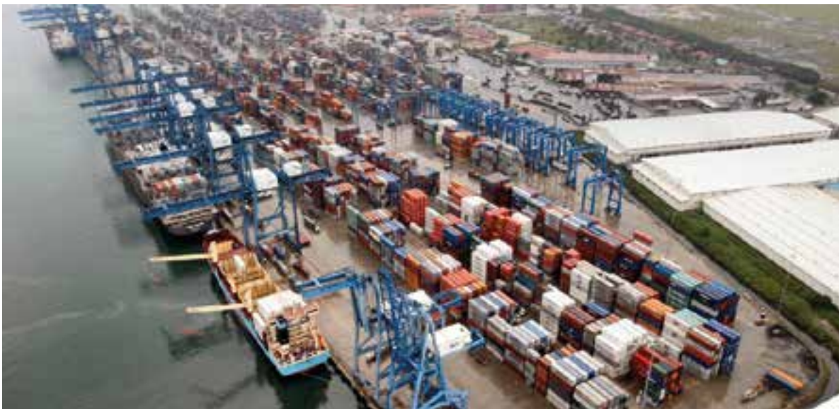
Tideworks recently completed integration and development work at Manzanillo International Terminal
