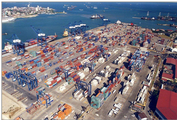
Manzanillo International Terminal (M.I.T.) – Colon, Panama
