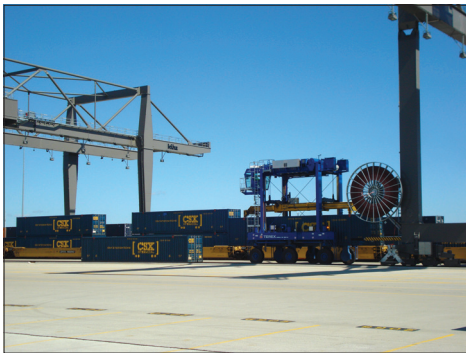
Tideworks IPro is now live at the new CSX terminal in Ohio
