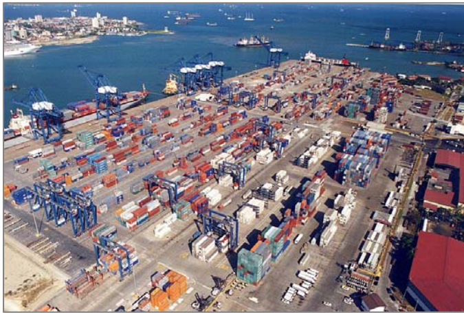
Manzanillo International Terminal (M.I.T.) – Colon, Panama
